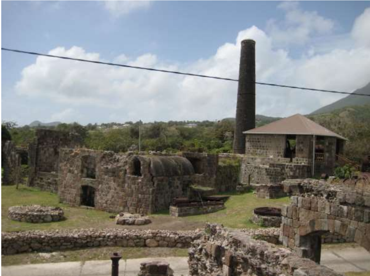
New River Estate works, Nevis, in 2017 A Fawcett boiler can just be seen on display to the right
